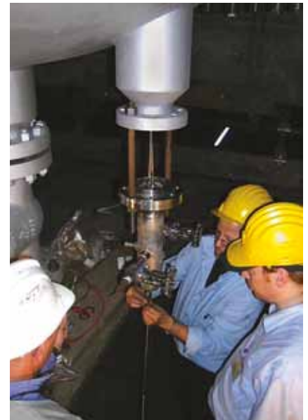
Installation of a multipoint thermocouple
