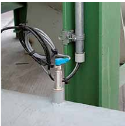
Monitoring of a supply pipework using compact thermometers and temperature switches
