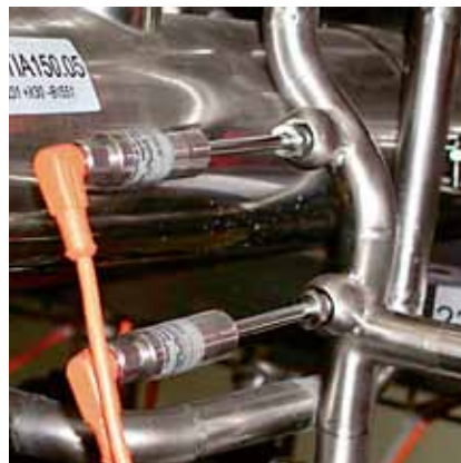
Monitoring of a supply pipework using compact thermometers and temperature switches
